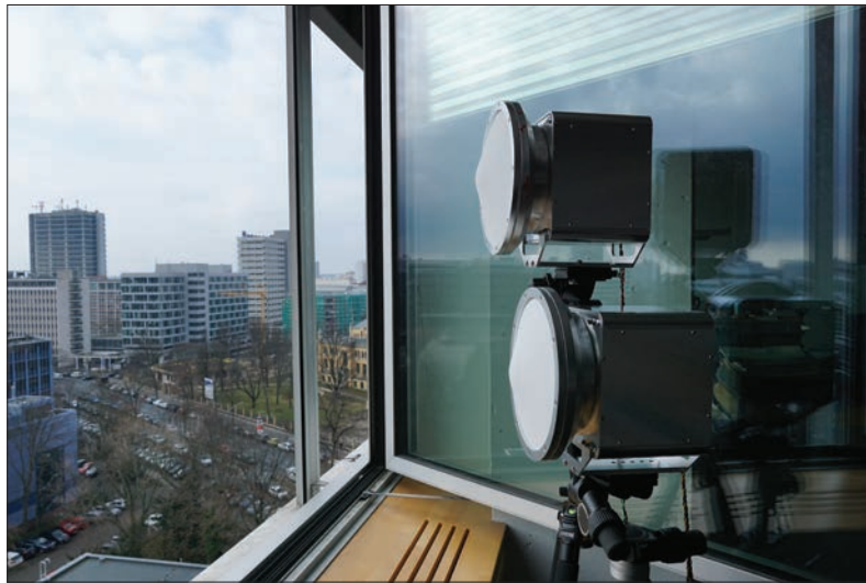
Figure 3. Photograph of the outdoor units at the receiver. The Berlin test site refers to a 500-m-long THz-wireless link between the campus of the Technical University of Berlin and the Fraunhofer Institute for Telecommunications, Heinrich Hertz Institute (HHI). This particular placement of two outdoor units corresponds to a PDM configuration.
